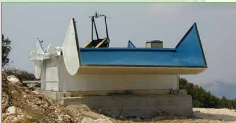
Figure 2.4a: The TAM inside its cylindrical dome
