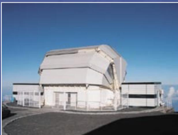
is located on Maui, Hawaii (Faulkes Telescope North) and the other is located in Siding Spring, Australia (Faulkes Telescope South). Each telescope stands 8 metres tall and has a 2 metre diameter primary mirror and a field of view up to 30 arcminutes in diameter.
